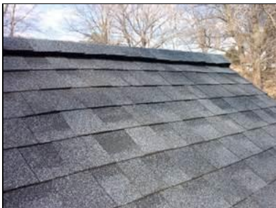
1.2 Item 1(Picture) Ridge Vent
