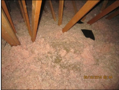
8.1 Item 1(Picture) Attic Insulation
