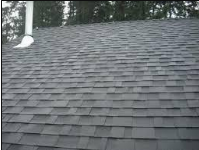
1.0 Item 1(Picture) Right Rear Roof
